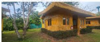
SINGLE ENSUITE ROOMS
